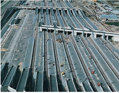
Channel Tunnel Terminal, UK
