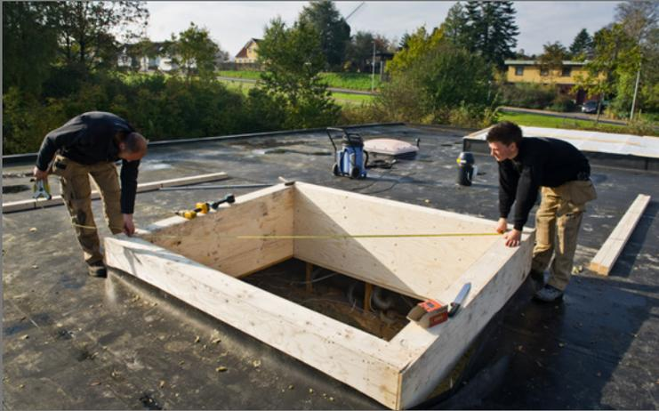
To support an easy installation process, the sub-construction needs to accommodate the very specific system installation. Modular skylights require an accurate fixed-dimension substructure. Likewise, the strength of the sub-construction needs to be calculated from project to project, based on the building design and application size.
