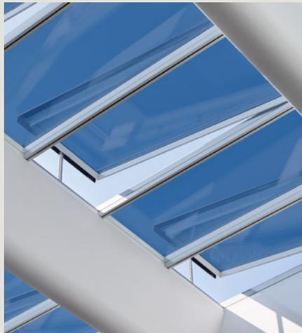
Glazing with electrochrome glass in intermediate state.
