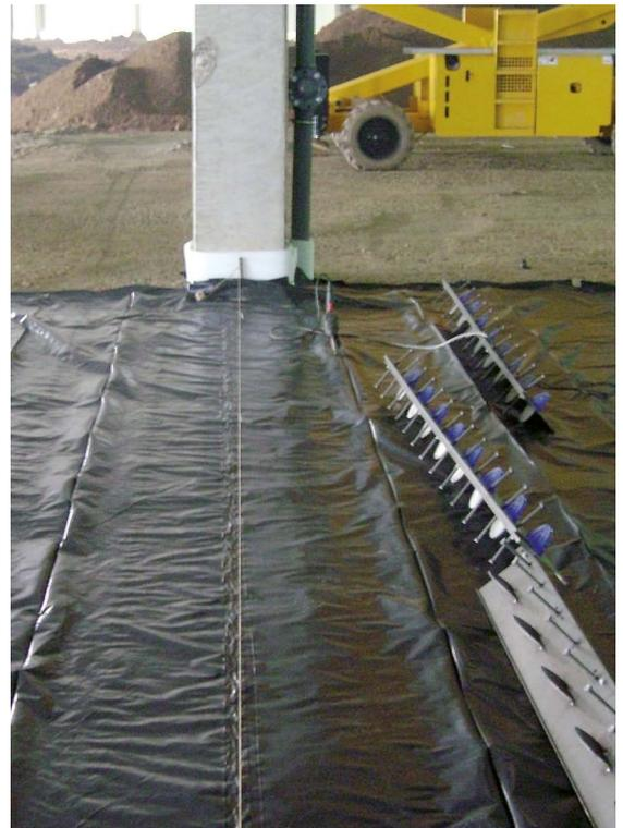
2. The joints are placed in the correct position according to the string line, and the height is adjusted. The height should be verified by laser level or similar at both ends, and the joint should be set vertical using a spirit level which can be placed across the top edges.
