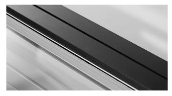
Aluminum cladding parts are treated with a scratch resistant powder coating. Here the cladding between two modules.
