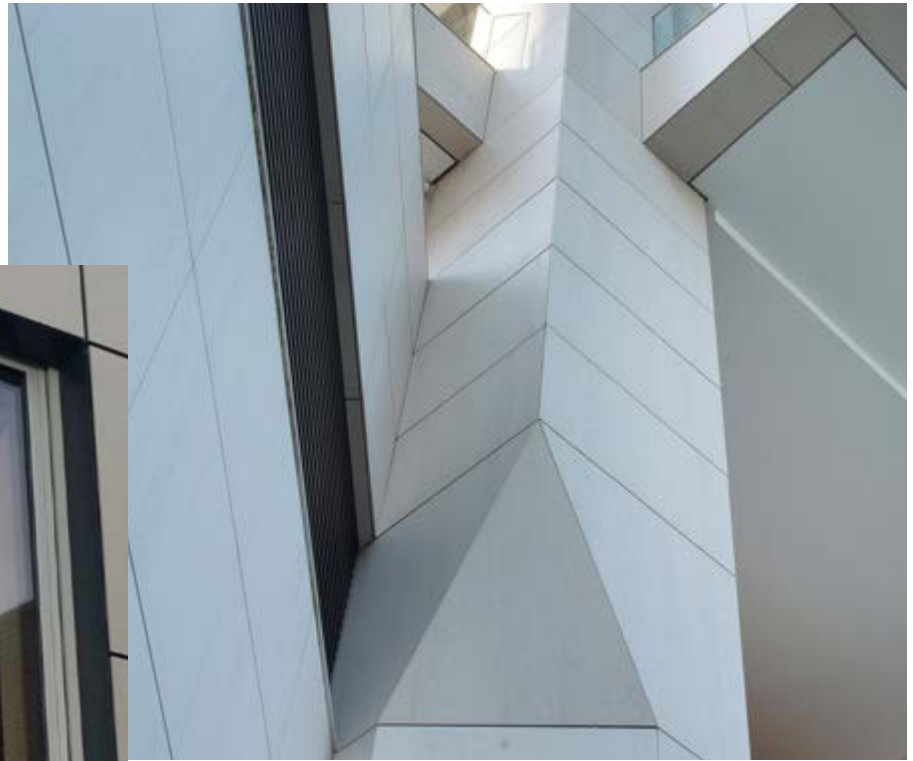
Cap Ferrat Building. Rio de Janeiro, Brasilien
