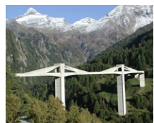
Ganter Bridge (CH)
