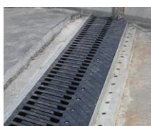
Sliding finger joints
