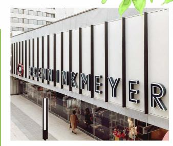
1969 Realisation of the first small facade project: C&A Brenninkmeyer in Leverkusen, Germany very simple cladding with unformed panels
