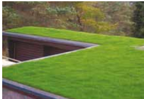
Extensive Green Roof 95kg/m 2 @ 5m Double-span
