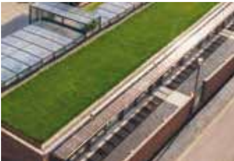
Intensive Green Roof 500kg/m 2 @2.5m double-span 250kg/m 2 @3.5m double-span
