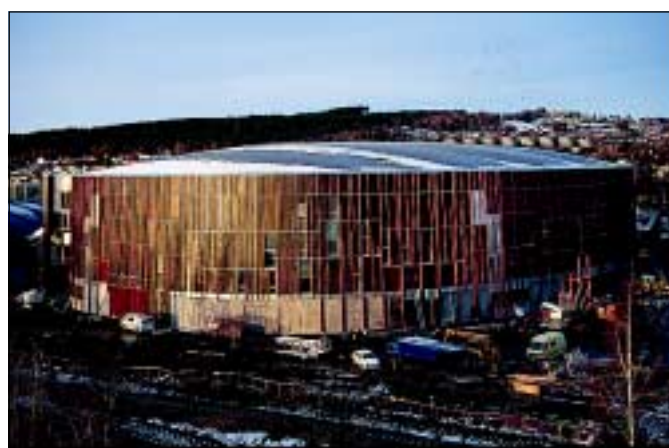
Hamar OL-amfi, Nordlyshallen
