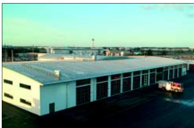
Brandstation Öst, bana 3, Arlanda
